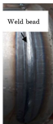
Fig. 1. Element of the gas tank under study.
